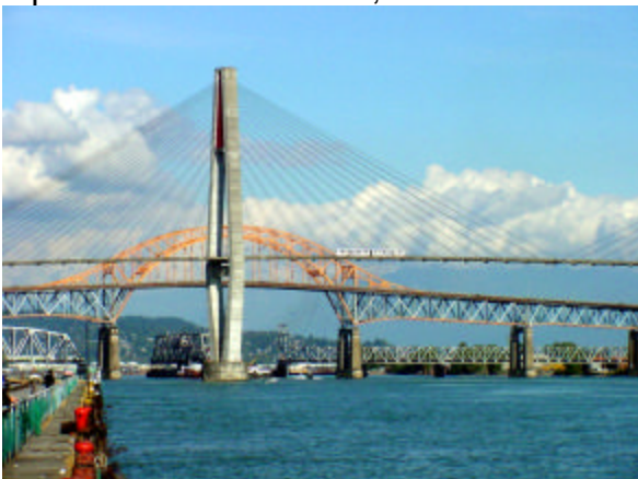
Skytrain Bridge over the Fraser, Dave Emery
